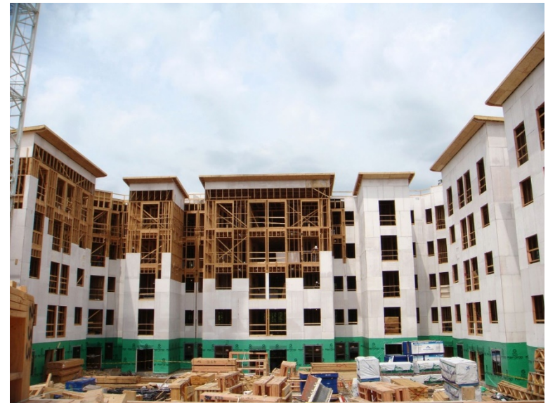
Exterior walls, Type III Construction The Varsity, University of Maryland, College Park, MD
