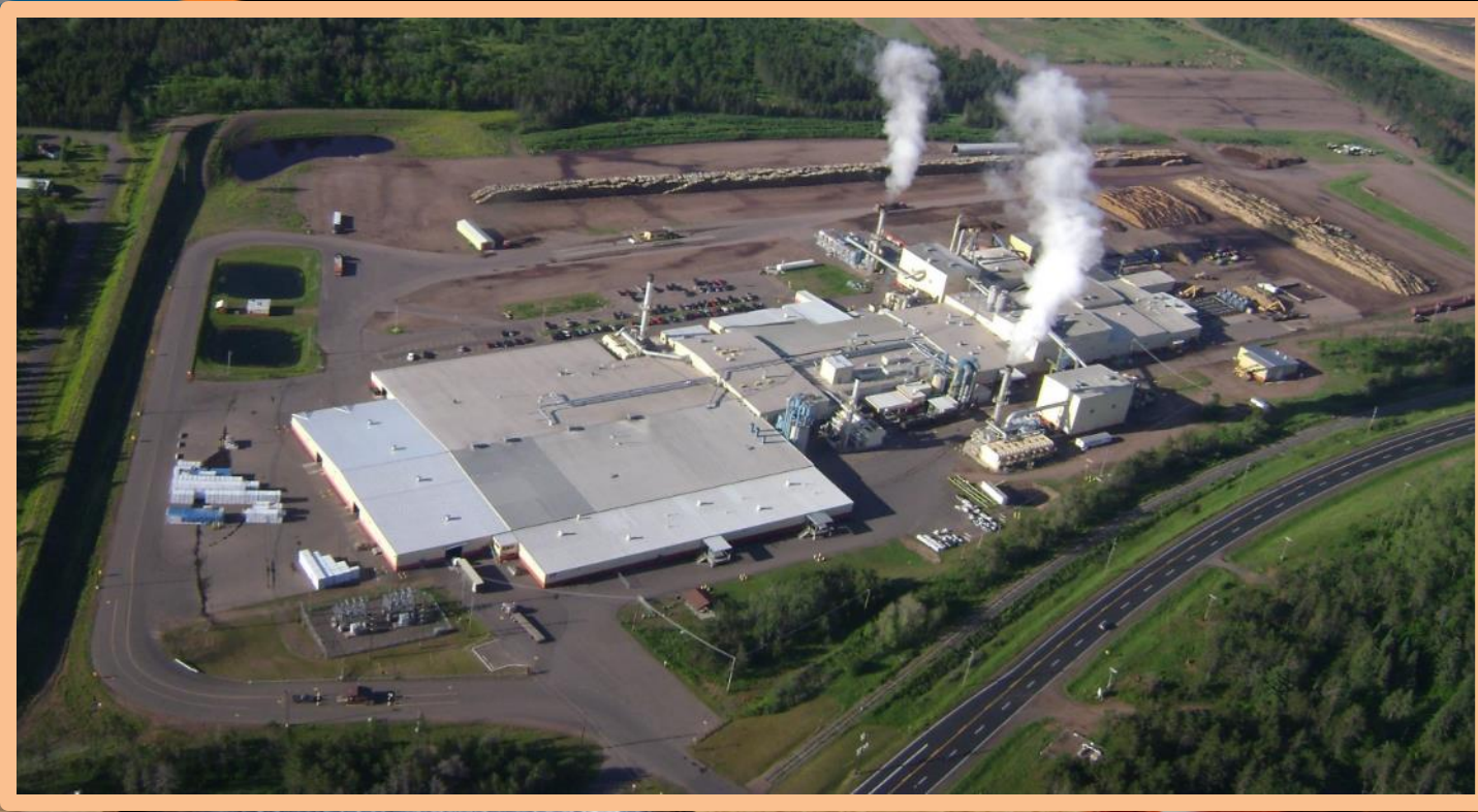
Plant Overview - LP Hayward
