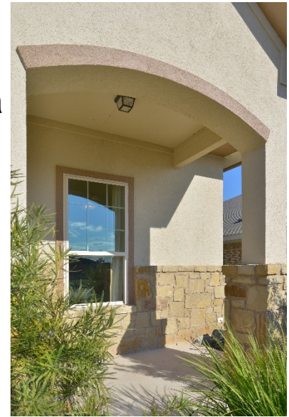
LP ArmorStrand single family house, San Antonio, TX
